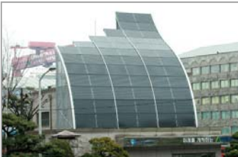
• Photovoltaic power generator in Ulsan shipyard
