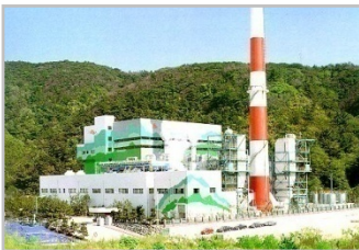
• Waste Incineration Plant
