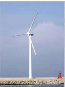
• 1.65MW wind turbine in the Ulsan shipyard
